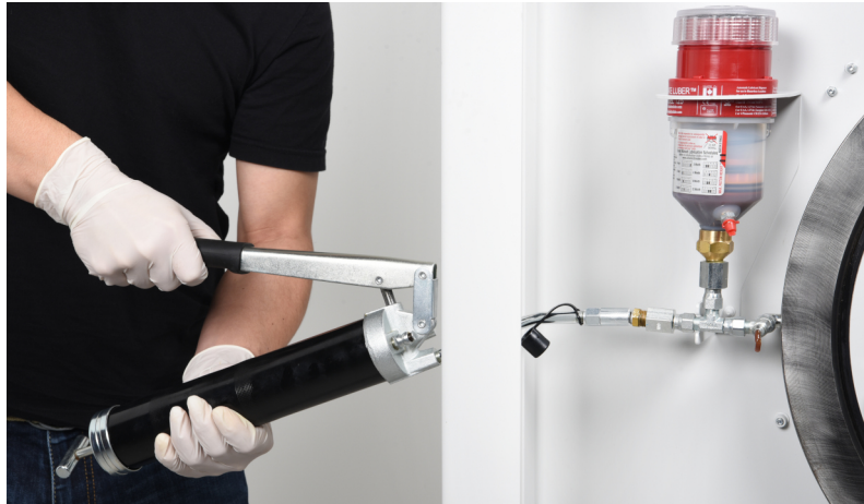
Figure 73. Pumping grease into the slewing bearing grease fitting.
